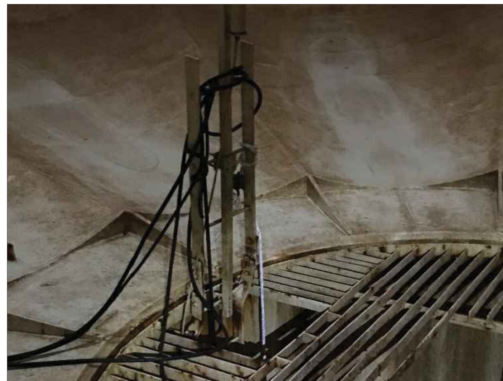
Figure 31. Interior Riser Ladder The rails have been spliced just above the grating and have been installed such that the ladder curves to one side to be more centrally located within the grating opening.
