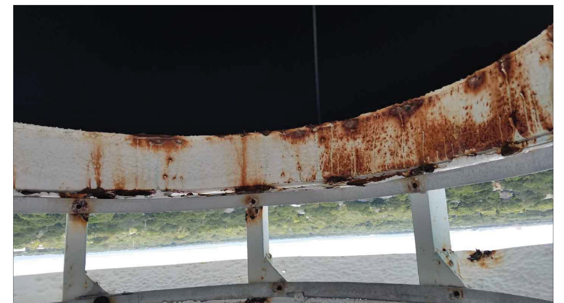
Figure 9. Top of Bowl Vent Repair corrosion on bowl vent and replace missing insect screen
