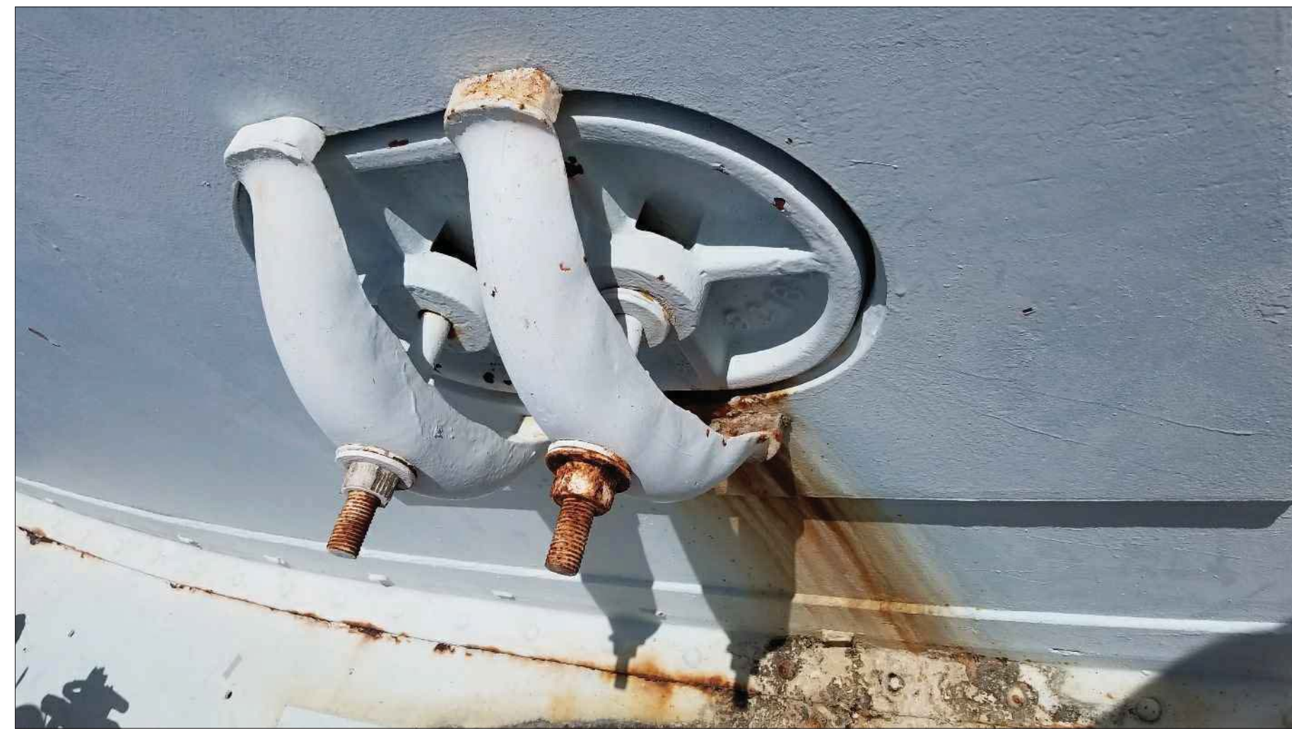
Figure 11. Exterior Bowl Access Portal Repair corrosion on bowl access portal hardware
