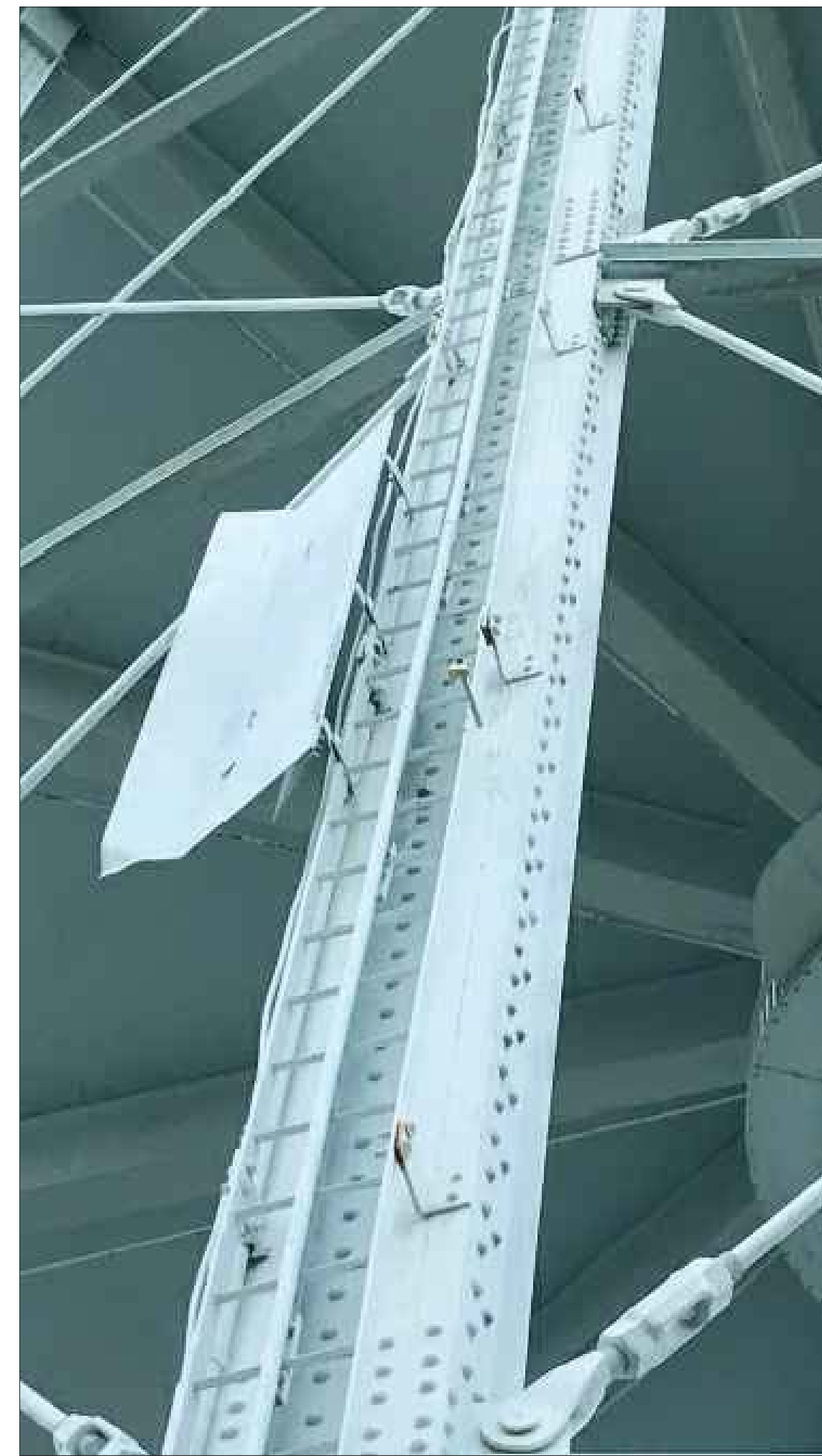
Figure 28. Exterior Outer Riser Ladder
