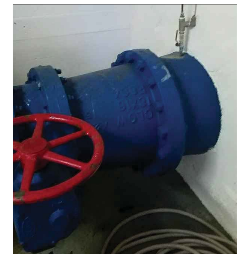
Figure 25b. Isolation Valves Remove and replace Isolation Valves
