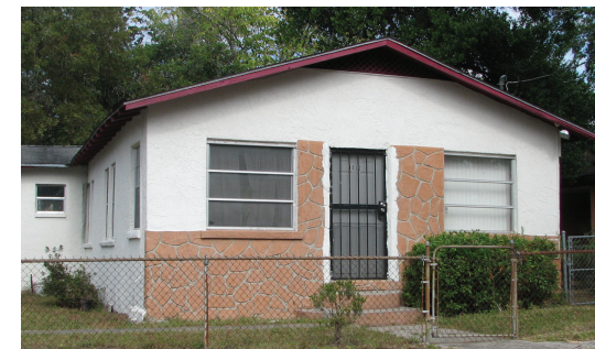
House at 3612 Shadowlawn was brought into code compliance.
