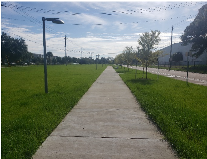
Figure 4.R: Images of Sidewalk Conditions
