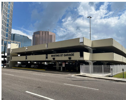
Whiting Street Garage
