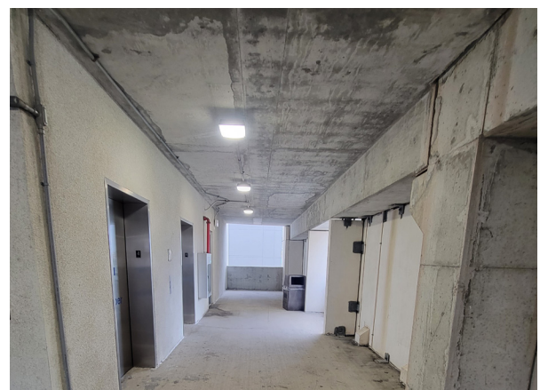
Northwest Elevator Bay
