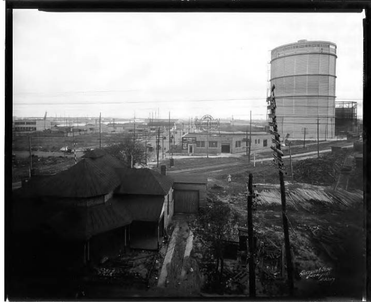
5 th Ave & 13 th St. – Tampa Gas Co. & Turner Music Co. Warehouse 1927 (Downtown CRA)
