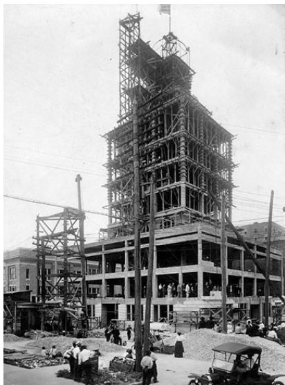
City Hall under construction in 1915.
