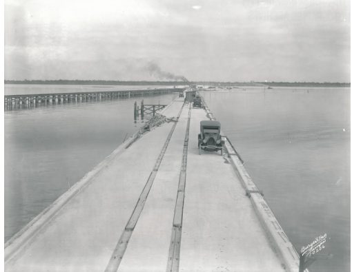
The Gandy Bridge under construction over Old Tampa Bay on December 17, 1923.
