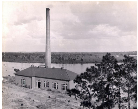
In 1924, construction began on a new water treatment plant on the Hillsborough River near 30th Street, which is pictured here.
