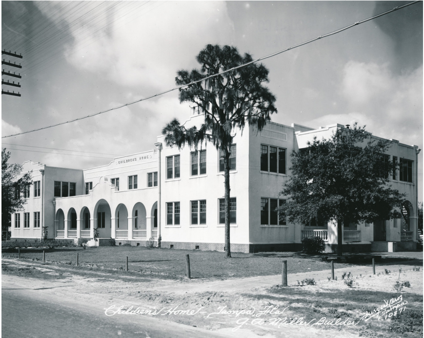
View of the Children's Home at 3302 Florida Avenue. This building still stands 100 years later in 2024.
