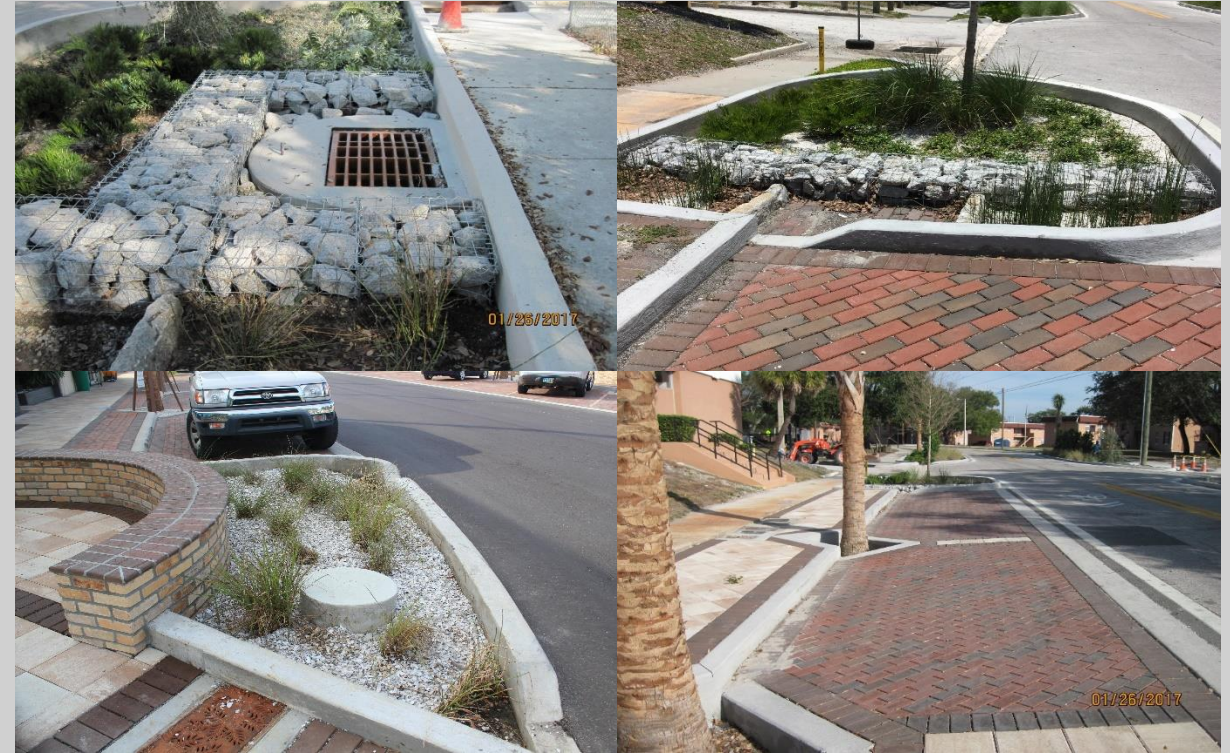
Pervious pavers for on-street parking (Scott Street) Low impact development features at bulb-outs
