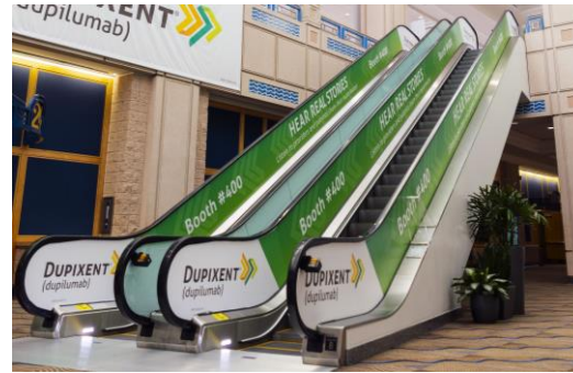
Escalators from 1 st Floor to 2 nd Floor
