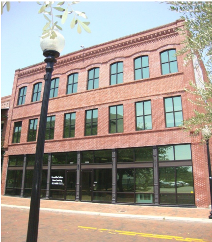
C.C. Burns Furniture Store Building 1207 N. Franklin Street constructed 1910
