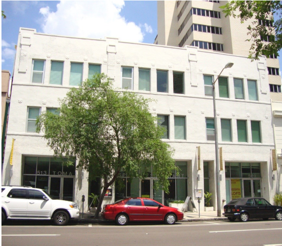
Spain Restaurant 509-513 N. Tampa Street constructed 1921
