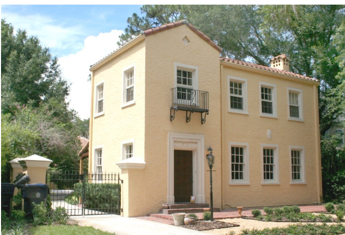
4505 W. Beach Park Drive, constructed 1925
