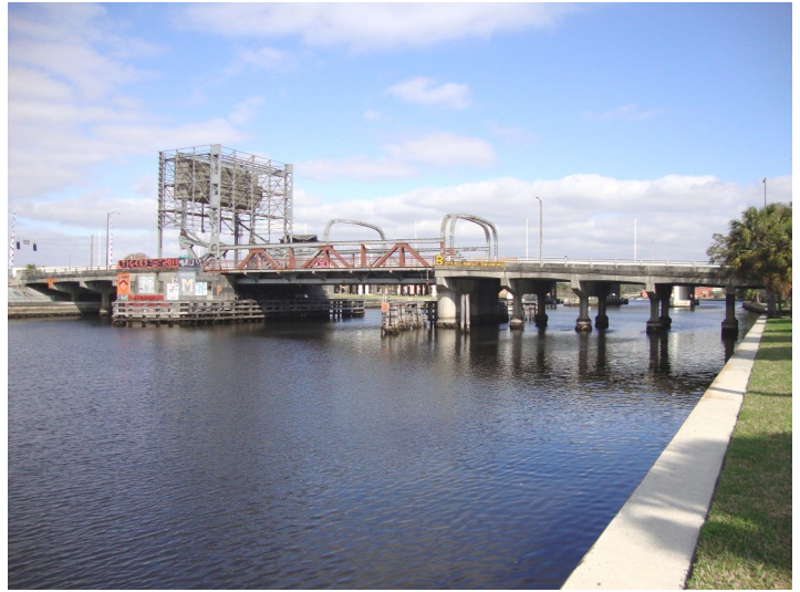
Fortune Taylor (Laurel Street) Bridge, constructed 1927
