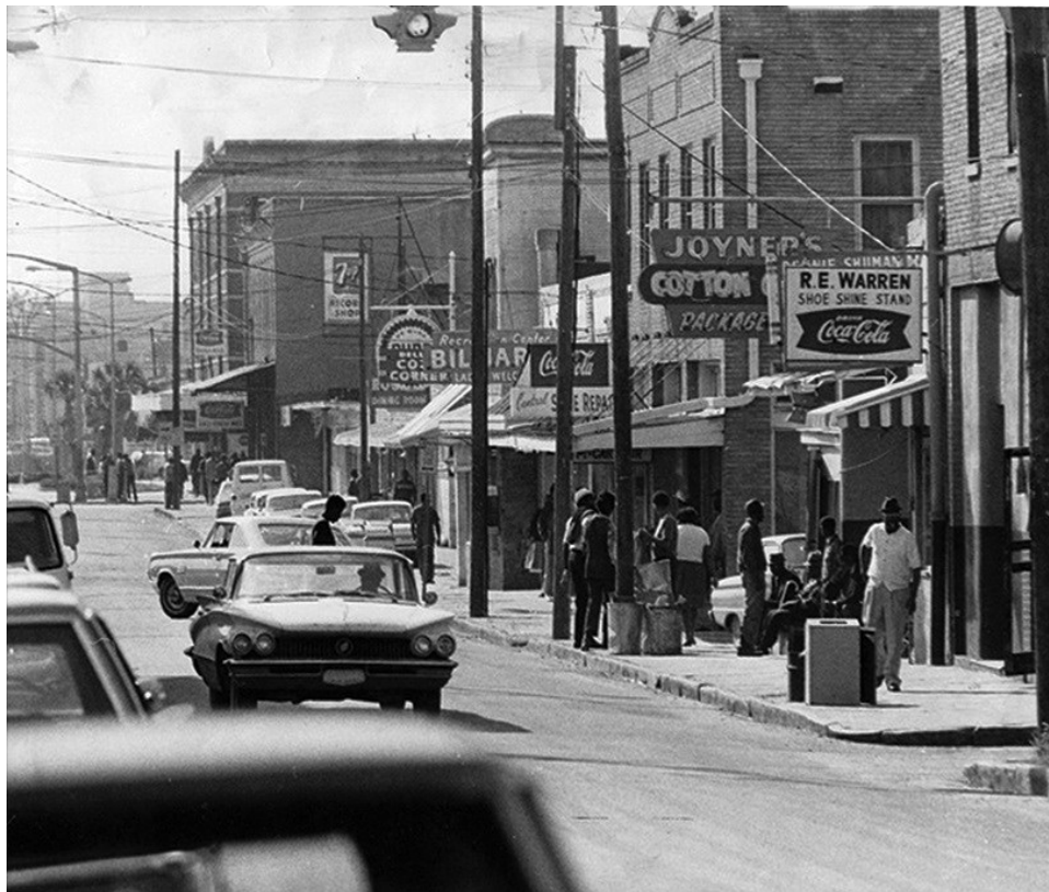
Central Avenue, 1960s
