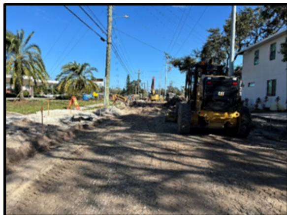
Himes Avenue – Installation of Water and Box Culvert
