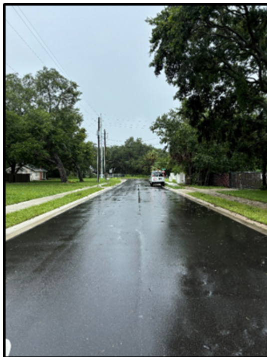
Averill Road – Complete Restoration
