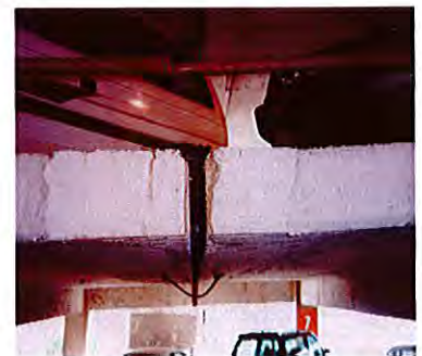
JOINT ON SUPPORTED FLOOR SLAB
