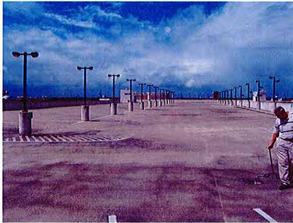
ROOF LEVEL OVERVIEW
