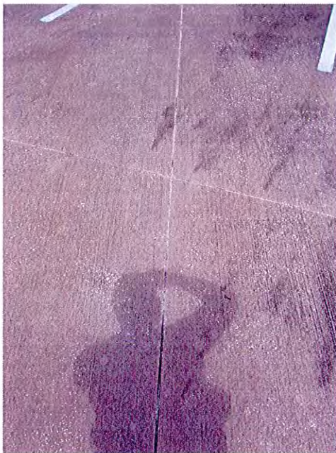
SAWN TOPPING JOINTS
