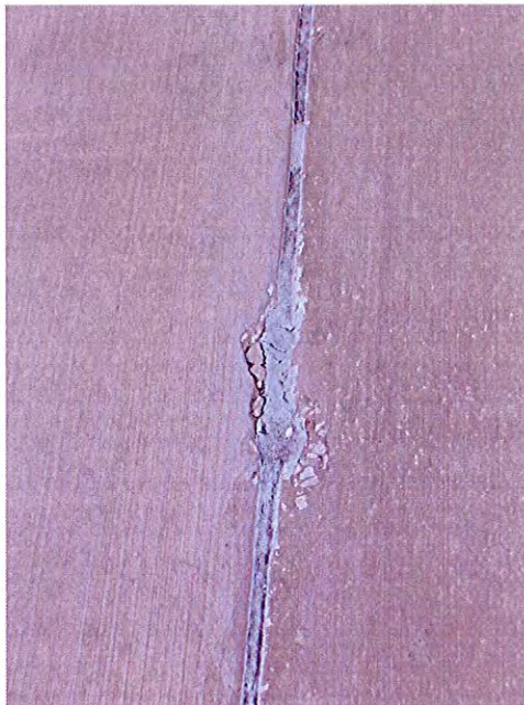
JOINT EDGE AND SEALANT DETERIORATION
