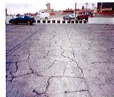
CRACKING
