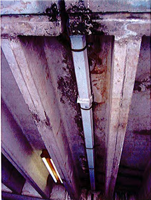
PONDING WATER AND THROUGH-SLAB LEAKS
