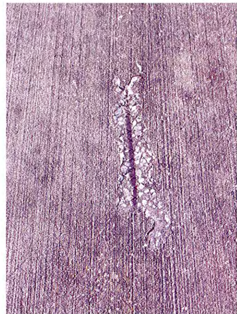
SHALLOW DELAMINATION
