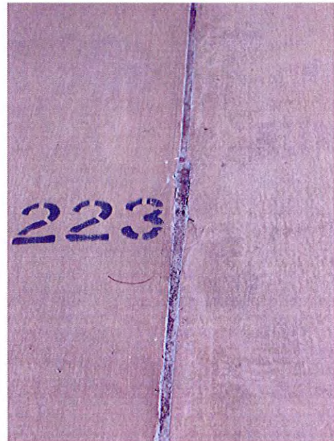
JOINT EDGE AND SEALANT DETERIORATION
