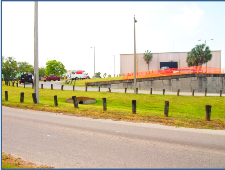
Transfer Station Photo No. 2B-28
