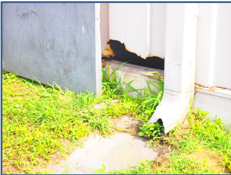
Transfer Station Photo No. 2B-33
