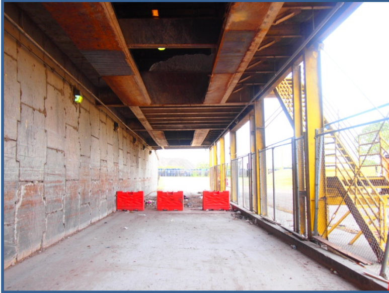
Transfer Station Photo No. 2B-59
