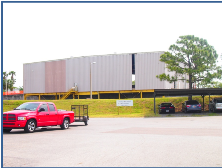
Transfer Station Photo No. 2B-23
