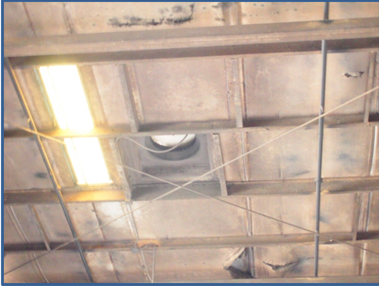
Transfer Station Photo No. 2B-42
