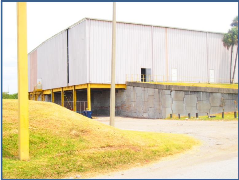
Transfer Station Photo No. 2B-25
