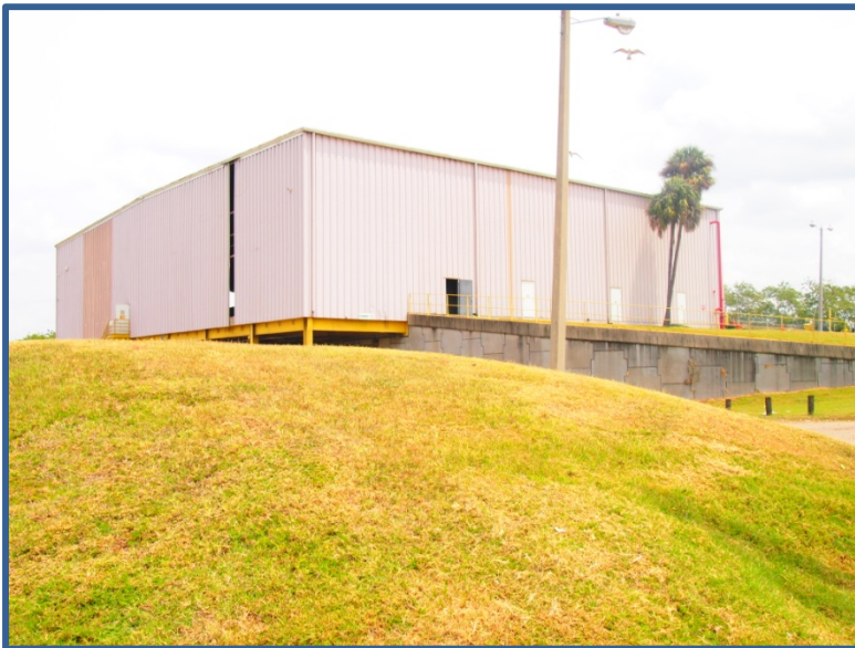
Transfer Station Photo No. 2B-31
