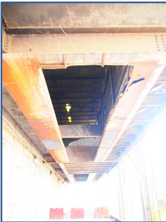
Transfer Station Photo No. 2B-60
