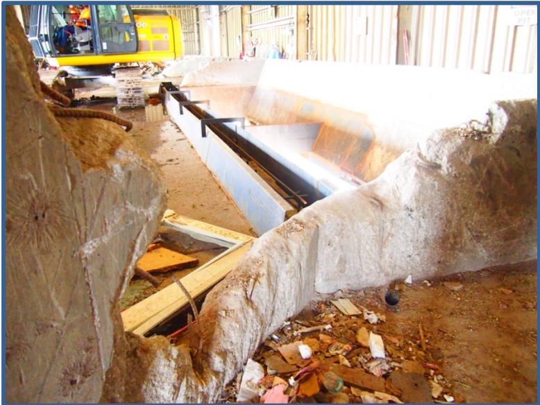
Transfer Station Photo No. 2B-54
