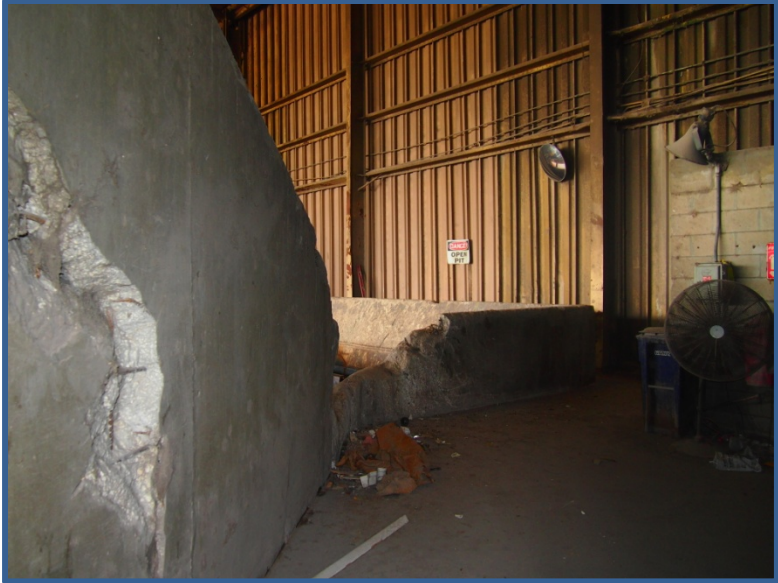
Transfer Station Photo No. 2B-53
