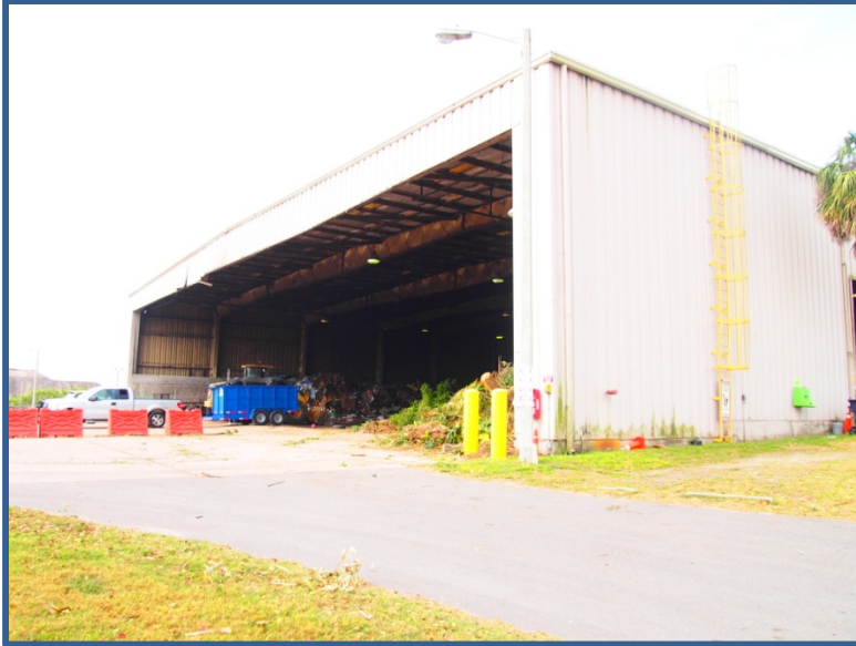
Transfer Station Photo No. 2B-30
