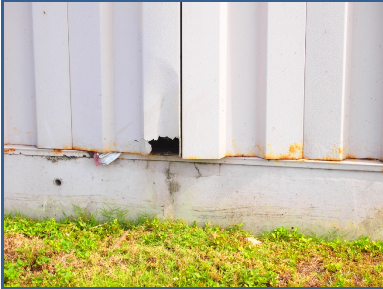
Transfer Station Photo No. 2B-32
