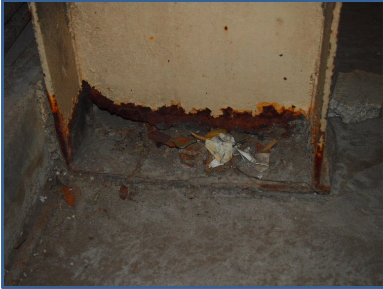
Transfer Station Photo No. 2B-44
