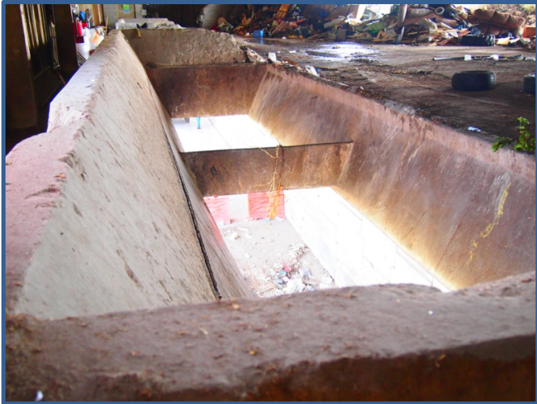
Transfer Station Photo No. 2B-52
