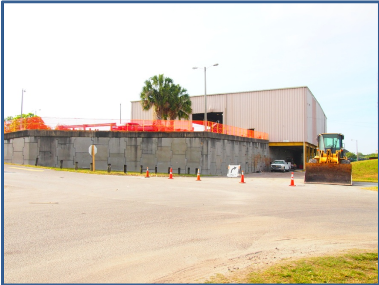
Transfer Station Photo No. 2B-24
