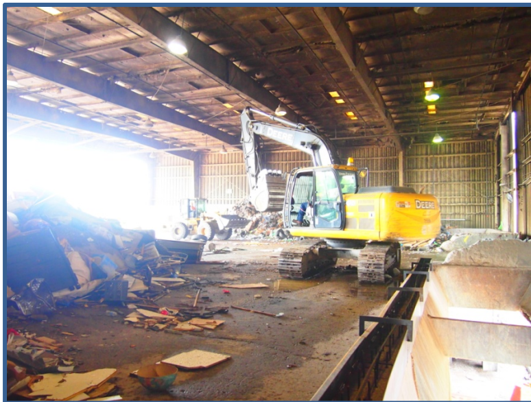
Transfer Station Photo No. 2B-41
