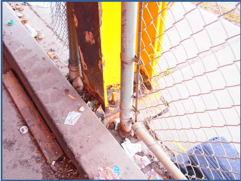
Transfer Station Photo No. 2B-27
