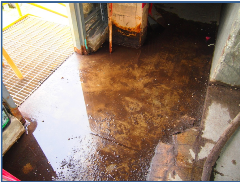
Transfer Station Photo No. 2B-43
