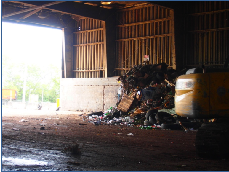
Transfer Station Photo No. 2B-38
