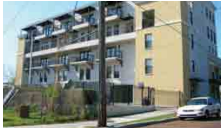
Rear yard conflicts between mixed use residential building on 4 th Avenue and outdoor storage uses south of Ybor CRA 2.
