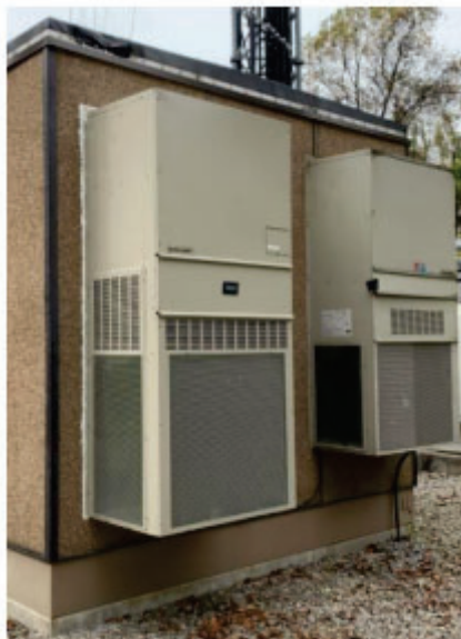
Figure 3-11: Packaged Wall Mounted AC Unit
