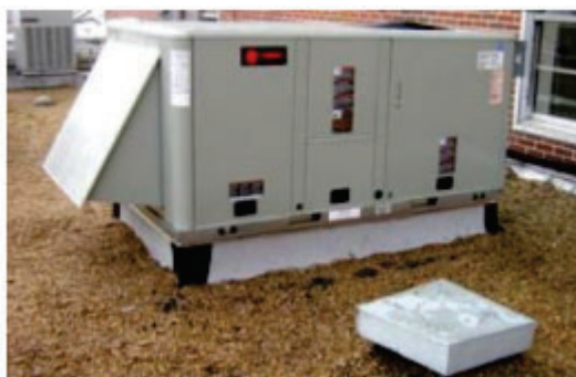
Figure 3-12: Packaged Rooftop AC Unit
